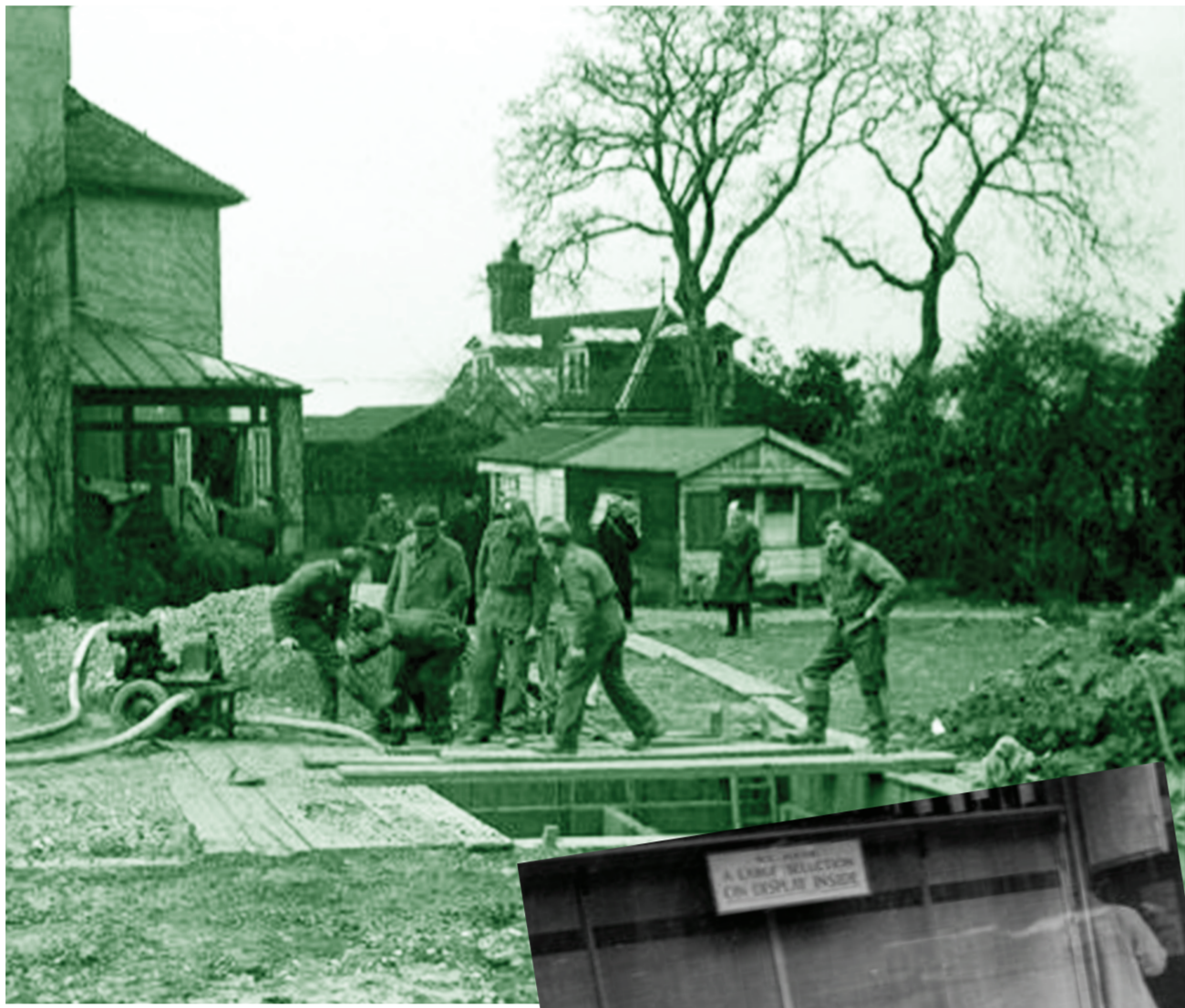
Garden of Wick House, Sparrows Herne. Members of an army Bomb Disposal team pumping water from a bomb hole in order to reach the bomb and defuse it.
